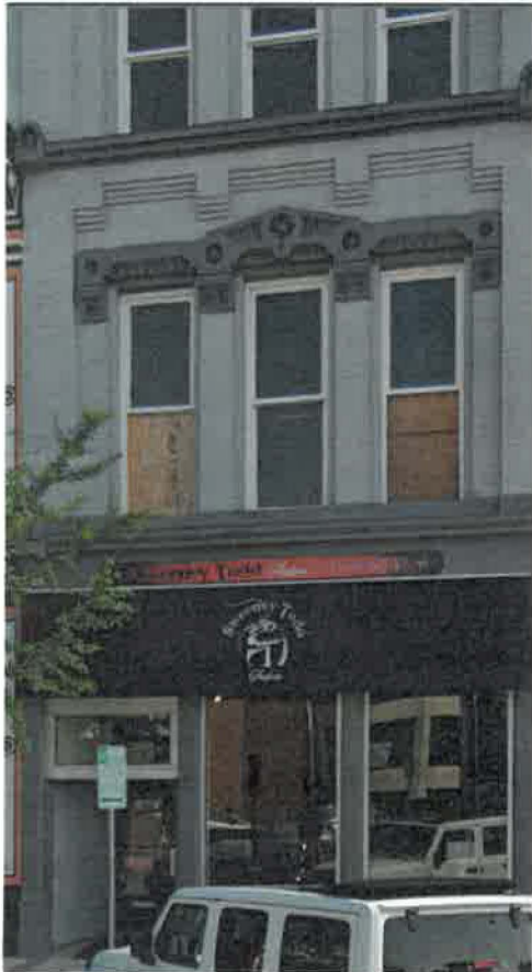
Current Exterior View (as of 6/25/25)
