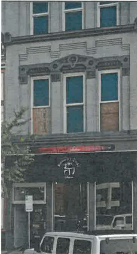
Current Exterior View (as of 6/25/25)
